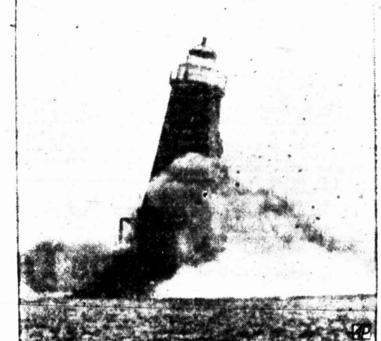
END OF A LIGHTHOUSE — Dynamic blast topples 150-year-old Bishop and Clerks Lighthouse, off Hyannisport, Mass., destroyed by Coast Guard lest it fall on fishermen.
