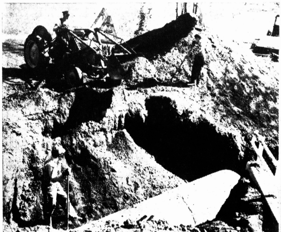
CITY CONTINUING WITH PAVING PROGRAM—A 36-inch culvert was being added to a ditch on 700 Blk. N. Russell Saturday prior to the paving of 700 and 800 blocks. City employees shown are Leo Jones, 625 N. Christy, tractor driver, and Pierce Walker, 608 N. Dwight, standing in ditch. Watching is Riekey Schmidt, 801 N. Frost. (News Photo)
