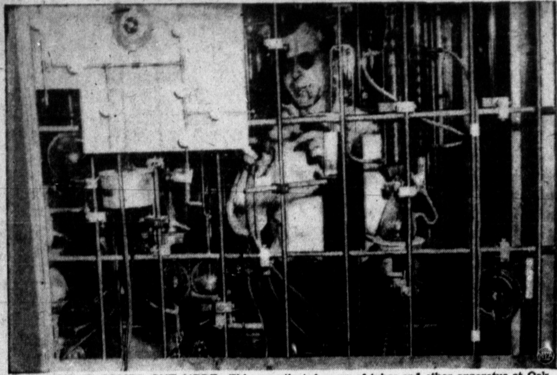
... AND IT COMES OUT HERE—This complicated array of tubes and other apparatus at Oak Ridge, Tenn., National Laboratory, merely siphons off one of the by-products of the big atomic pile. B. J. Massey is sealing off a tube of tritium, which has made its way through the man-made "jungle." This was one of the Oak Ridge operations shown to newspaper reporters and photographers for the first time, as they watched how the atomic pile "cooks" and processes radioactive isotopes for medical and industrial uses, as well as for atomic bomb production.
