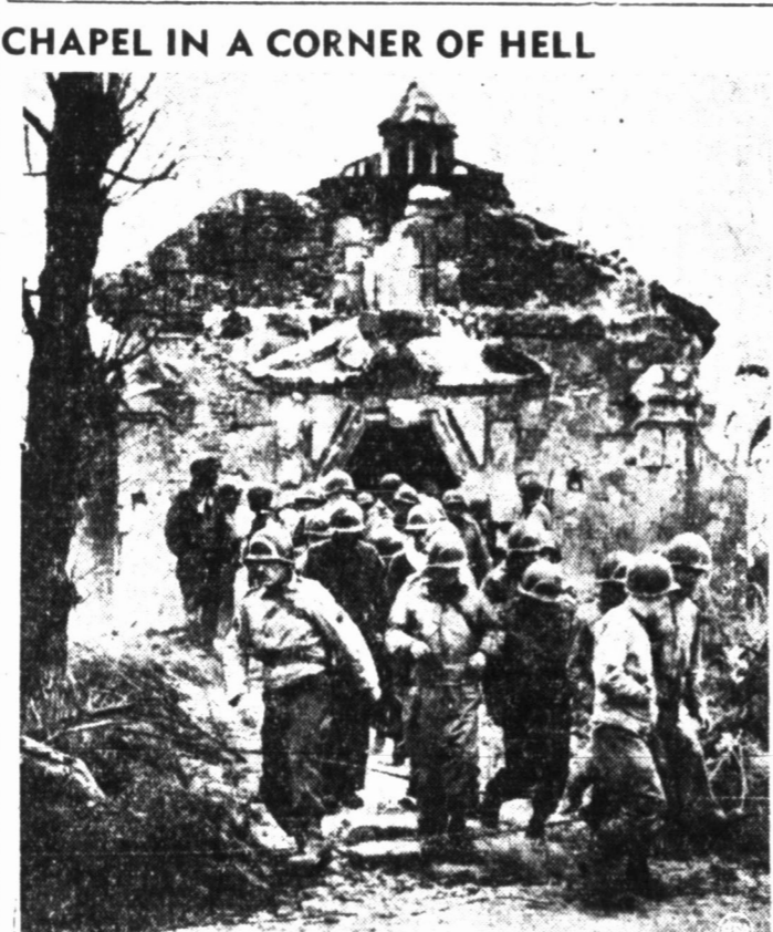
CHapel IN A CORNER OF HELL Its walls smashed and shell-pocked from the furious battles that raged around it, this little Norman chapel buried above provided religious services for Allied fighters. Ringing out above the din of war, the chapel bells summoned soldiers pictured above to worship.
