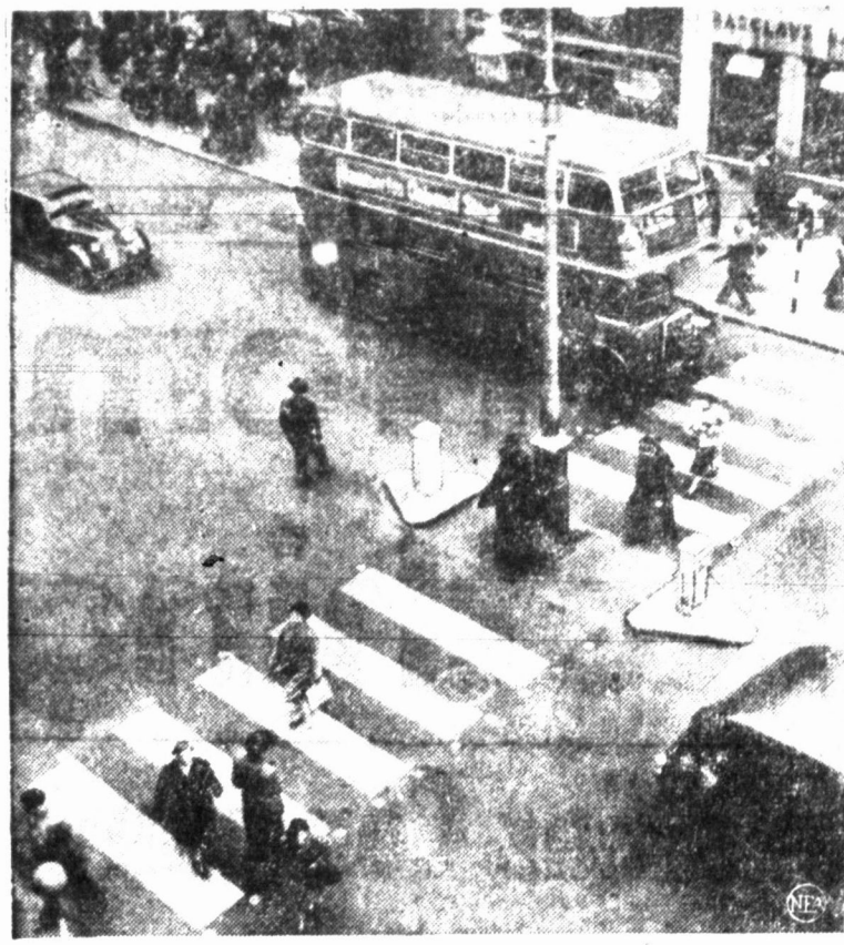
THE WAY IS BARRED —This "zebra-walk" of broad white bars across the pedestrian cross-walk is one of the giants England's Road Research Laboratory is using in working out safety measures for big-city traffic. The striped zone is reported not fully satisfactory as a safety measure.
