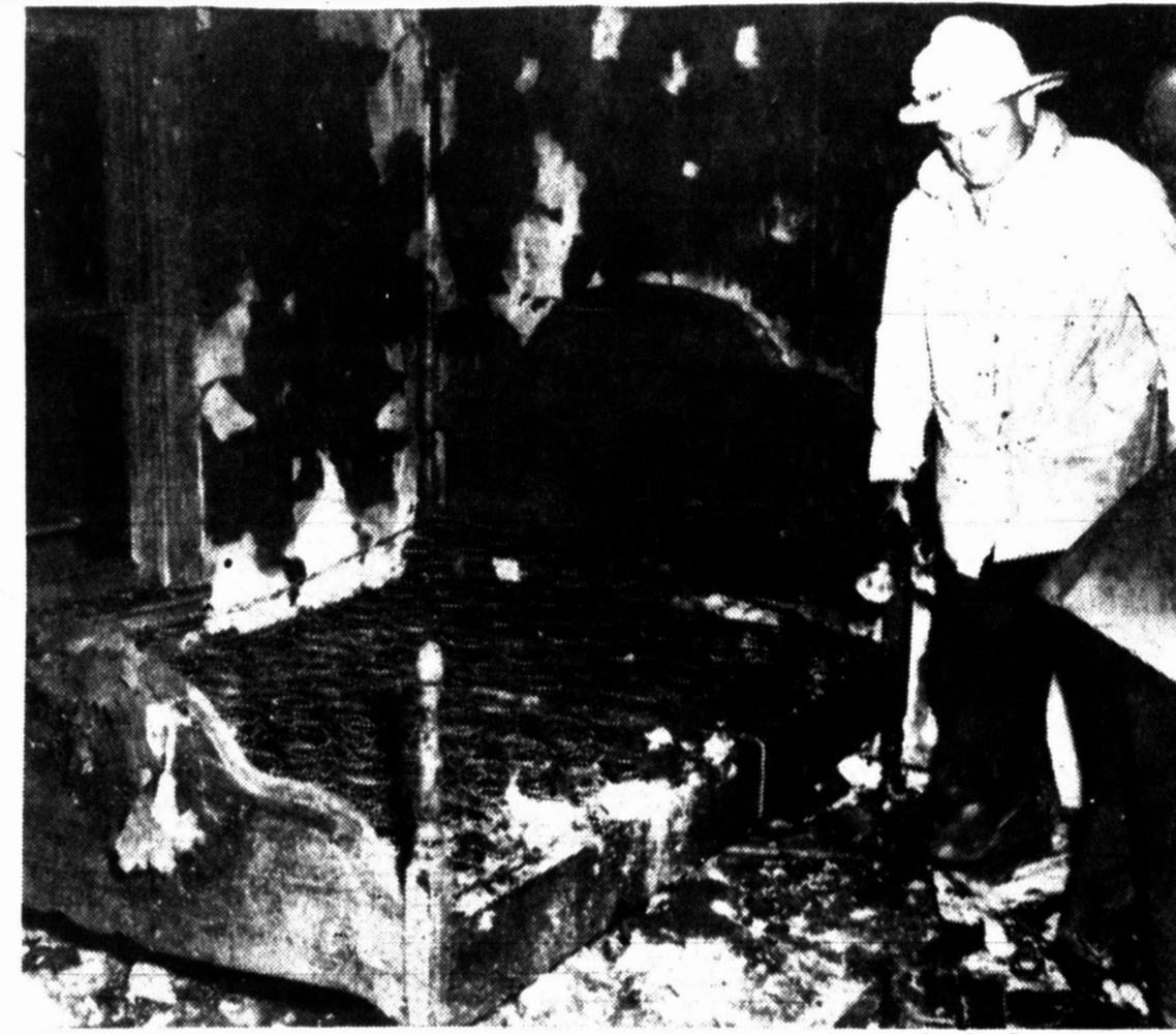
AFTERMATH — Fire Chief Ernest Winborne surveys damage caused by a fire Sunday at 634 E. Craven in which the interior of a house was destroyed. R. C. Owens, who was sleeping at the time of the fire, barely managed to escape without injury. Cause of the fire is believed to be from make-shift wiring. (News Photo)
