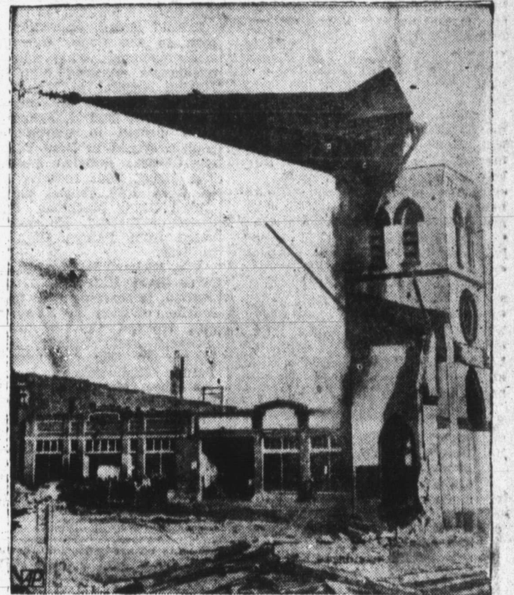
HEADING FOR THE GROUND —The wooden steeple of a 65-year-old Denver, Colo., church is caught in midair as workmen demolish structure to make way for business building.
