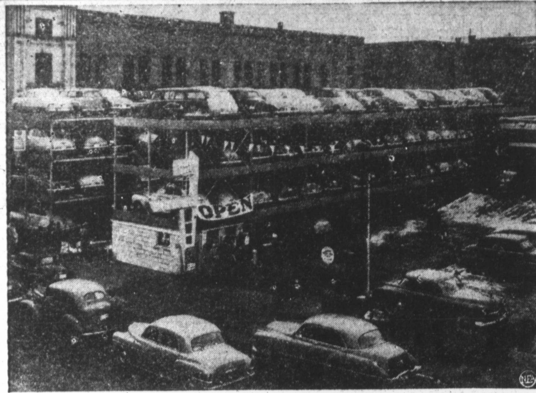
PIGEON-HOLE PARKING—Auto parking gets a big lift in Spokane, Wash., with the operation of this automatic parker which is half trolley and half elevator. Powered by special motors and controls, the car parker runs on a track in the middle corridor, lifts the auto to the desired level and deposits it in one of the "pigeon-holes."
