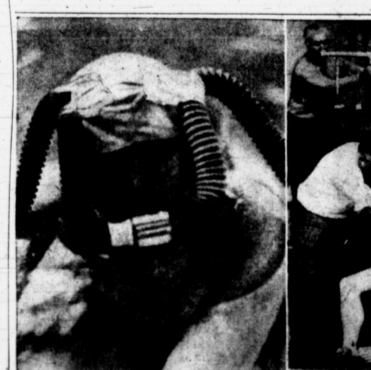
MAN FROM MARS?—No, the grotesque figure in the Illinois pool is John Marshall, wearing a rig devised by Dr. T. J. Curerton to study oxygen consumption. Right, Marshall rests after all-day swimming test. Dr. Curerton determines the heart response with a stethoscope. Technician Richard Gansten checks recovery blood pressures. Exhaled breath is collected in the canvas bags in the background, later is analyzed.
