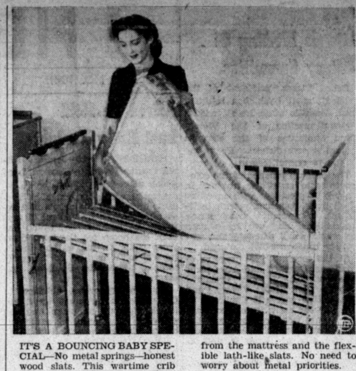
IT'S A BOUNCING BABY SPECIAL —No metal springs—honest wood slats. This wartime crib gets its comforting softness from the mattress and the flexible lath-like slats. No need to worry about metal priorities.
