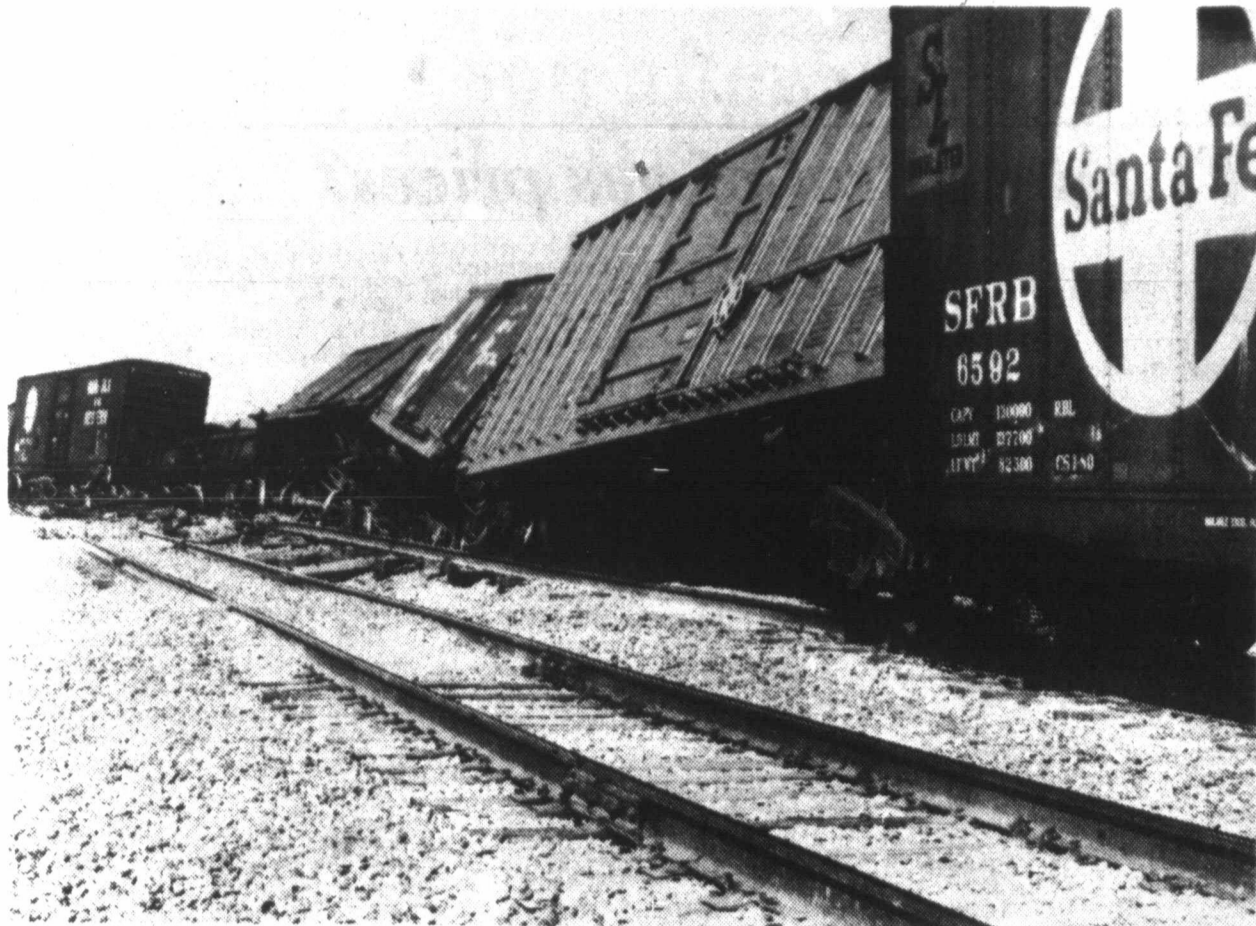
RAILCARS STAND at all angles along the railroad tracks between the Cabot Carbon Black plant and Ingersoll Rand where a 22-car derailment occurred Sunday evening. Santa Fe officials estimate damages in the accident to reach $133,000. Railroad employees were working through the night to clear the tracks for other trains. (Staff Photo)
