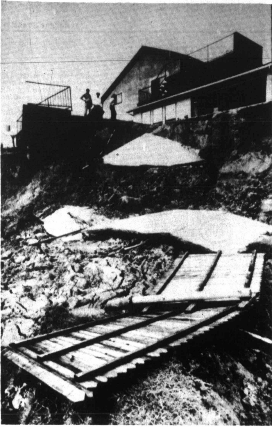
MUD SLIDES. This North Arlington house was evacuated Wednesday after mud slides left it perched precariously on a 30-foot cliff over the Trinity River bottom. One other house was also evacuated and no one was injured in the slides which began Monday afternoon as cracks in the back yards of the houses. (AP Laserphoto)
