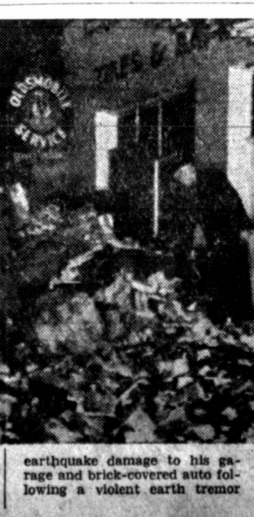
earthquake damage to his garage and brick-covered auto following a violent earth tremor
