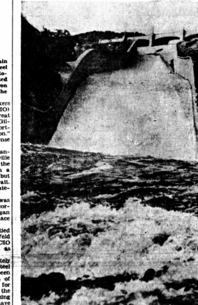
With water standing 2.52 feet above the spillway sill, a single gate was opened for test purposes recently and the man-made channel, 50 feet wide and 715 feet long, got its first wetting since the dam was built in 1916 near El Paso, Texas.
