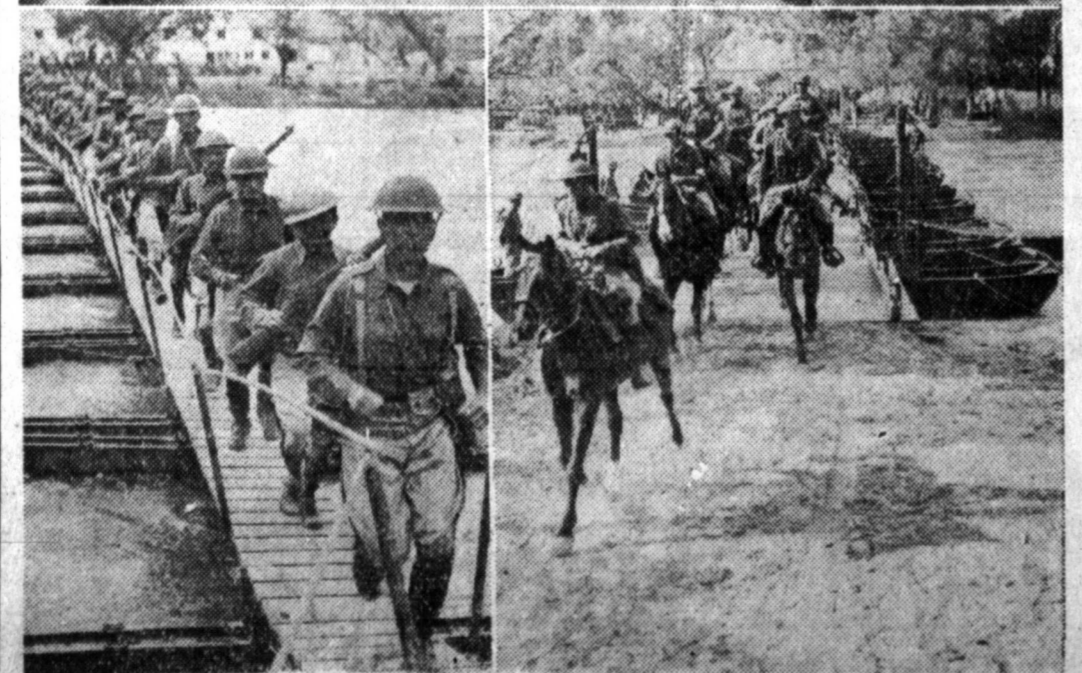
In a demonstration of speed and efficiency an 8th Engineers squadron strings a pontoon bridge across swollen Rio Grande river near Radium Springs, Tex., above, for a river crossing exercise in which the 12th Cavalry, bottom left, and right, was able to start crossing the river within 10 minutes of their arrival and the start of operations. In the top photo an armored car is already aboard the section of bridge being floated into place.
