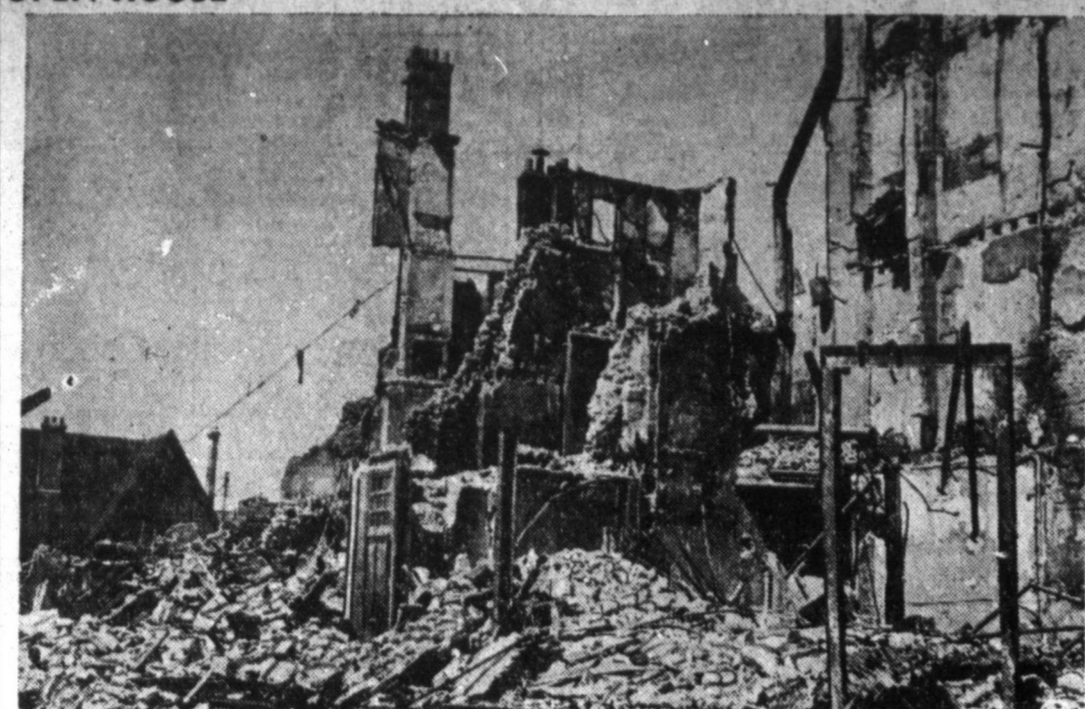
An ironical twist of fate left the door intact when this house in a French village was almost completely demolished by German bombing planes, according to French caption on this photo.
