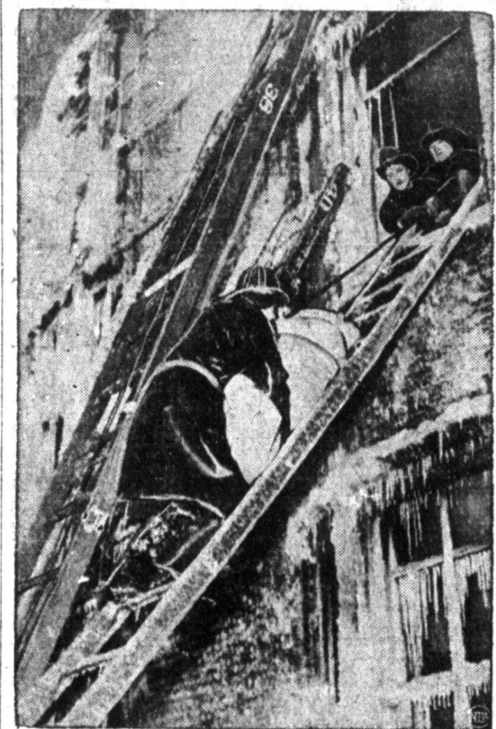
Trapped in an icy inferno, 18 persons died as flames raced up stairways and through halls of Marlborough apartment-hotel in Minneapolis after early morning basement explosion. Fireman on ladder, hampered by sub-zero weather, carries body of victim from ice-crusted ruins.
