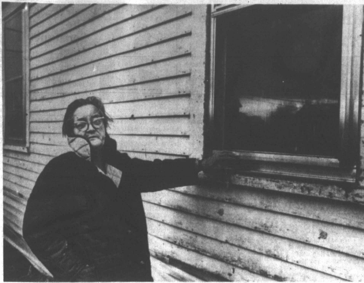
HOME WEATHERIZATION PROGRAM. Elsa Currier points to a storm window that was installed at her home in Chesterville, Maine, under the federally funded Home Weatherization Program. (AP Laserphoto)
