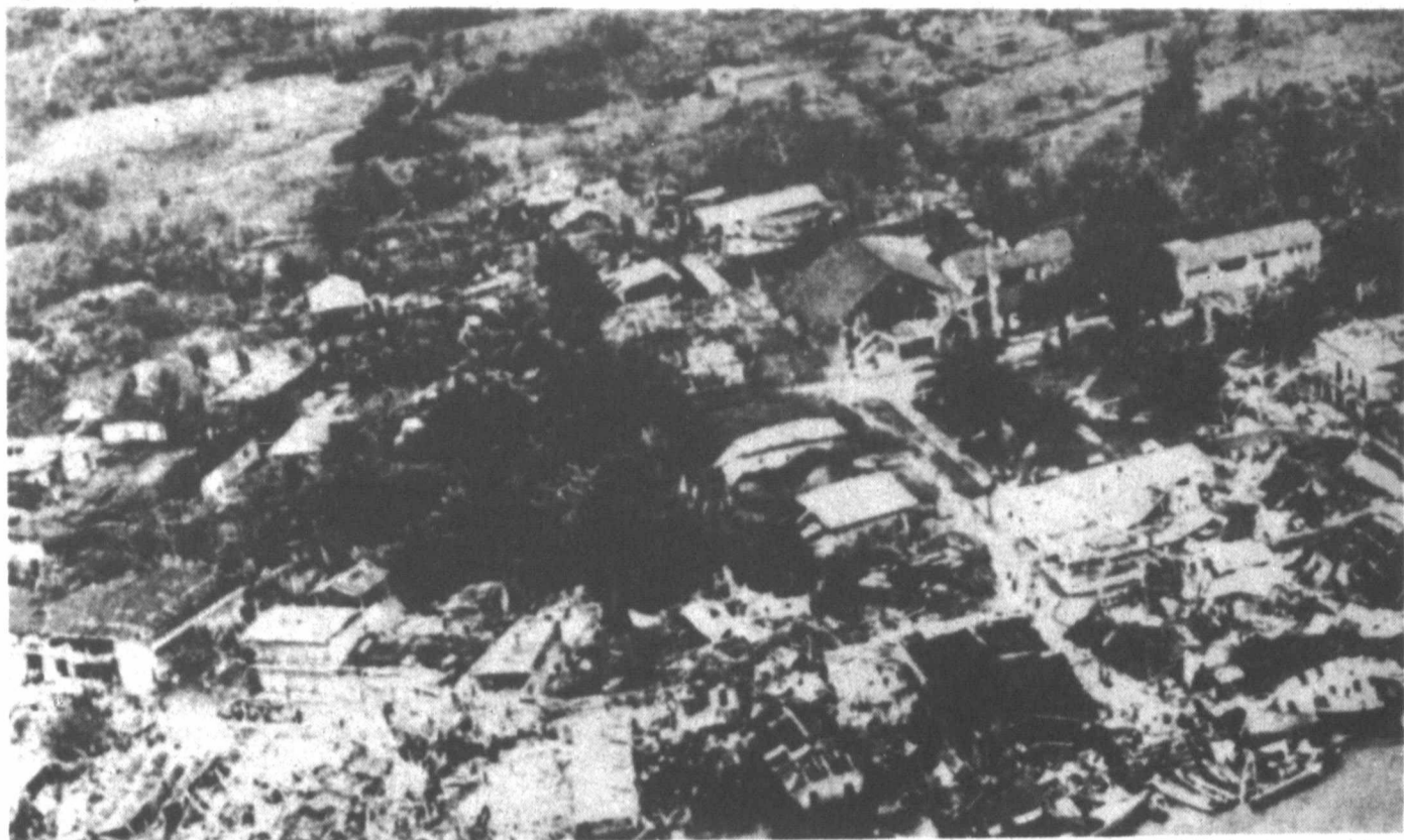
THIS AERIAL VIEW shows the Colombian Pacific coast town of Calico where 70 percent of the buildings in the fishing village of 4,000 were destroyed by an earthquake and resulting 10 foot
