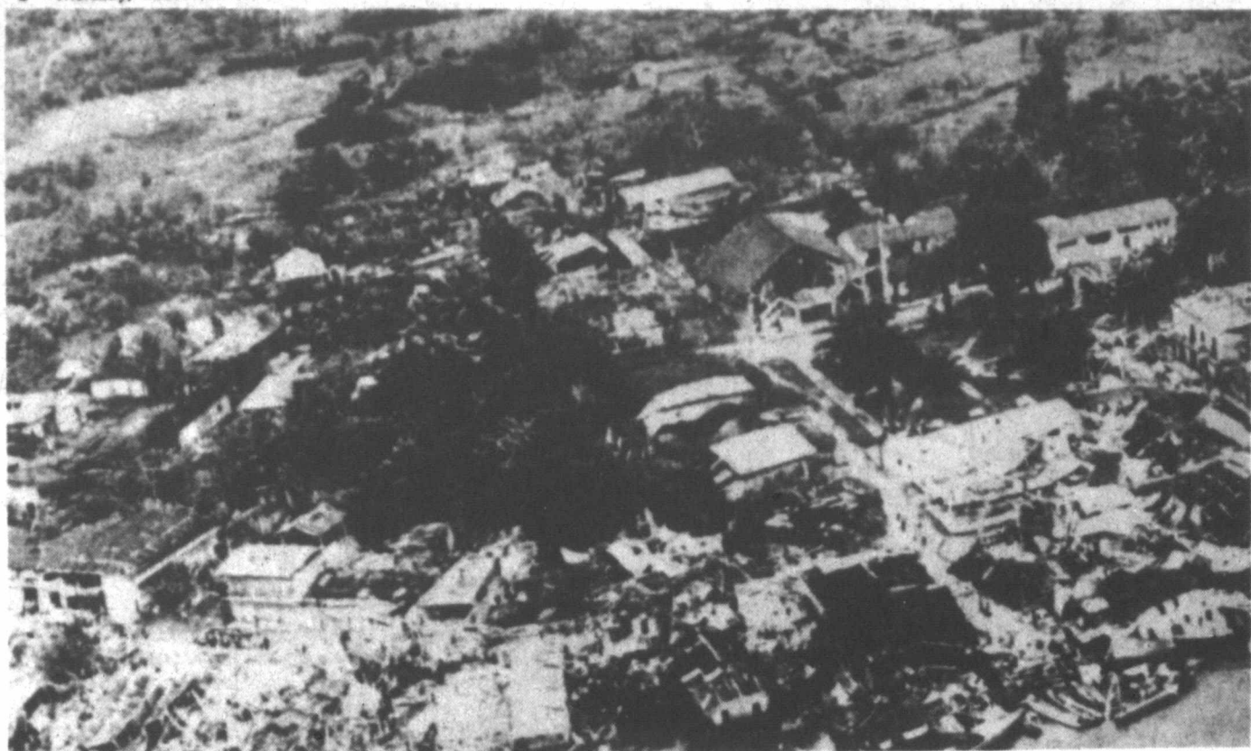
THIS AERIAL VIEW shows the Colombian-Pacific coast town of Calico where 70 percent of the buildings in the fishing village of 4,000 were destroyed by an earthquake and resulting 10 foot
