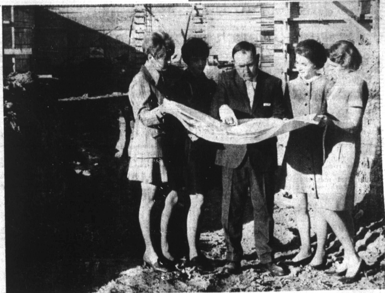
VIEW FROM THE GROUND UP — Four Junior Service League Provisionals examine plans and construction progress on Highland General Hospital's new wing with Wes Langham, hospital administrator. Provisionals pictured with Langham in front of the new wing's groundwork are from left, Mrs. Bill Neslage, Mrs. Paul Hartin, Mrs.
