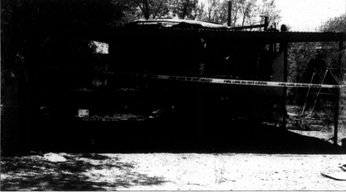
A fire reported at 4:09 a.m. Monday rendered this trailer home at 914 Denver uninhabitable for Larhonda Sue Willhite and her family. Keith Fisher, Pampa Fire Department fire marshal, said the cause of the fire is currently under investigation. A fund has been established for Willhite and her children who lost most of their possession in the fire. The fund is at First Bank Southwest in care of Sharon Strickland.
