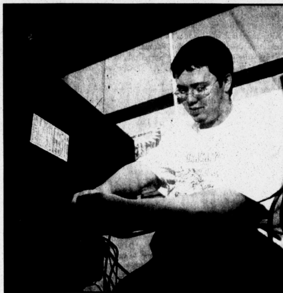
Cody Elliott checks wiring from solar panels to the electric motor that runs Pampa High School's solar car.
