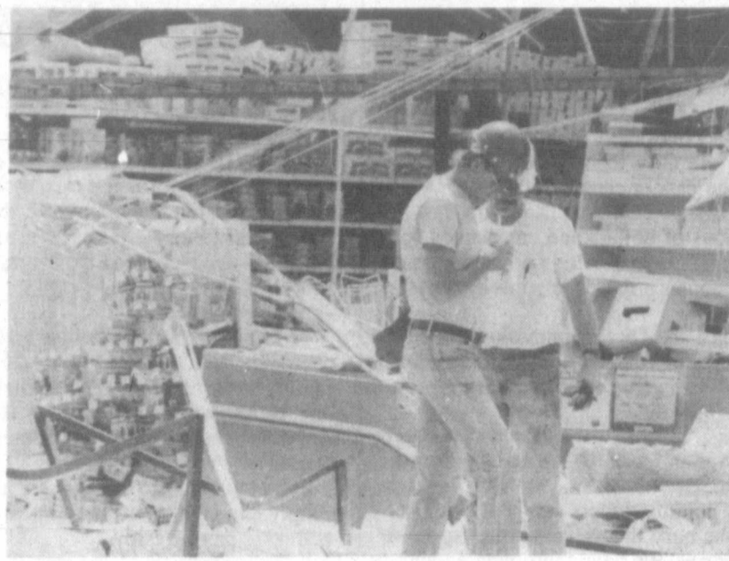
Workers look over debris in the Wal-Mart store in Colonial Heights, Va., on Saturday. Rescue workers and engineers are dismantling the building to look for missing people after a tornado struck Friday.
