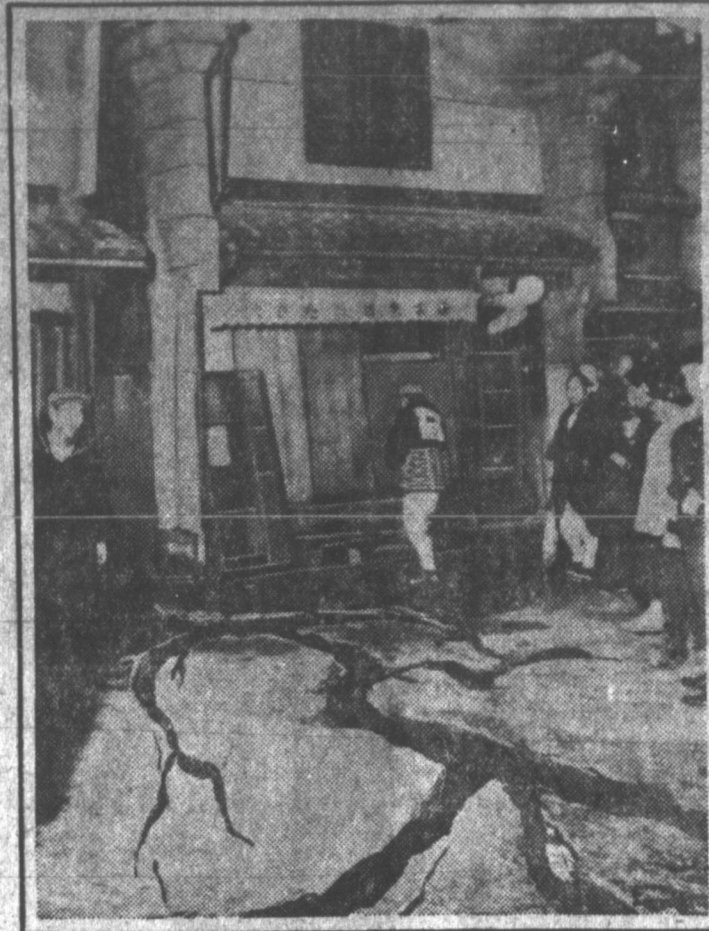
—NEA, Tokio Bureau A tremor which rocked the central part of Japan on March 7, demolished several towns and claimed more than 2000 lives. This picture taken at Osaka, shows the great cracks rent in the earth by the quake. It clearly shows how difficult it is to construct buildings that will withstand Japanese quakes.
