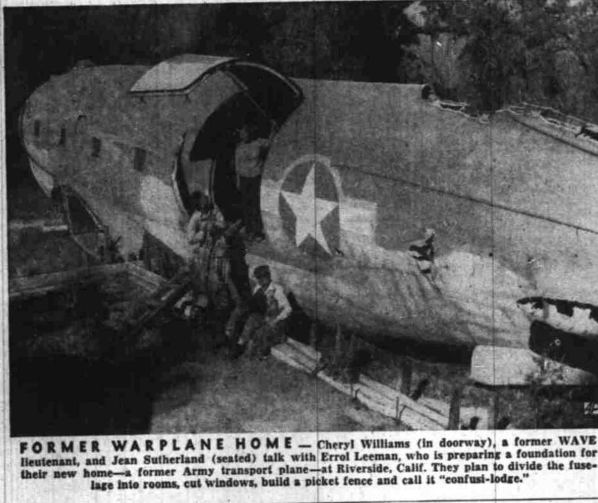
FORMER WARPLANE HOME — Cheryl Williams (in doorway), a former WAVE lieutenant, and Jean Sutherland (seated) talk with Errol Leeman, who is preparing a foundation for their new home—a former Army transport plane—at Riverside, Calif. They plan to divide the fuselage into rooms, cut windows, build a picket fence and call it "confut-lodge."
