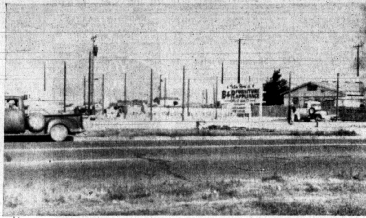
Work will be completed in about 6 wks.
