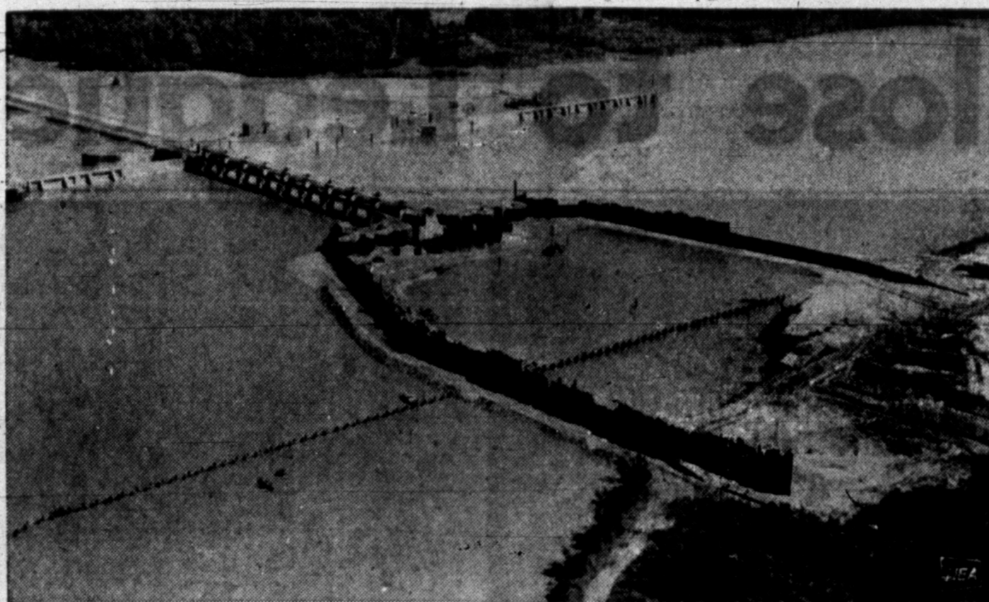
ARKANSAS RIVER LOCKS are taking shape in the U.S. Army Corps of Engineers project aimed at permitting barge transportation along more than 400 miles of inland waterways, besides providing flood control and hydroelectric power. This aerial view shows the lock and dam just below Little Rock, Ark., one of 17 such locks and dams to be built between Desha County, Ark., and Catoosa, Okla., at a cost of $1.2 billion. This particular job, typical of the others to be done, should be finished late in 1968. The construction is by Dravo Corporation of Pittsburgh, Pa.
