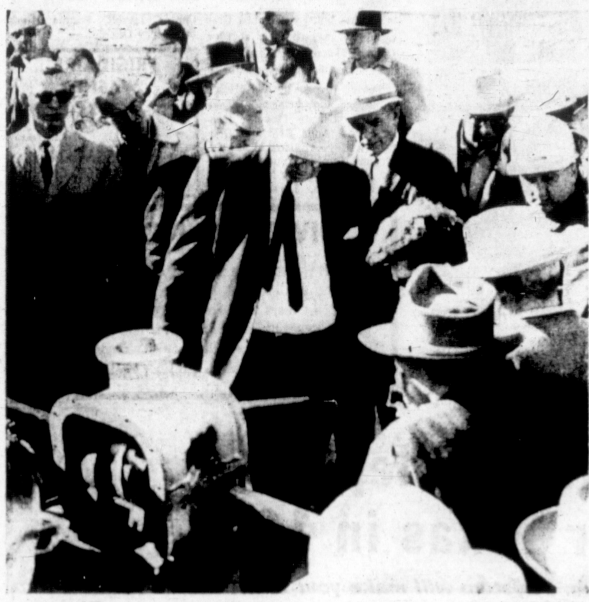
DEMONSTRATION — More than 200 oil men representing nine states attended a demonstration Tuesday afternoon in the Top O' Texas rodeo arena of a revolutionary gate valve that can be installed without interrupting the flow or operation of a pipe line. The valve was designed and built by C. L. Thompson, 435 Starkweather, who is standing nearest the valve and telling oil men about his invention. Thompson told the spectators that no production date has been established for the new valve but that it will be marketed by the Thompson Mark A-1 Valve company.
