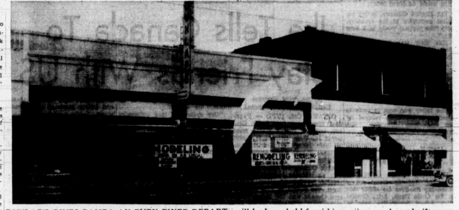
DUNLAP'S GIVES PAMPA AN EVEN FINER DÉPARTMENT STORE — Dunlap's is remodeling and enlarging to provide more complete and more convenient shopping for Pampa. The enlarged store will include the second story of the Dunlap Building, which will be connected with the present store by a modern elevator and staircase. This new addition will contain the complete ladies, girls and infants' departments. On the mezzanine floor selections in all departments.
