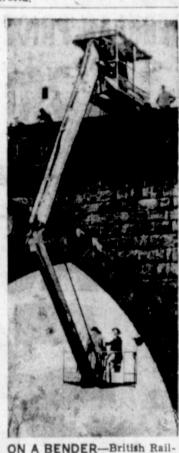
ON A BENDER-British Raillems in maintenance of their high-level bridges and viaducts, designed this "bender" to help their workmen. The device has two arms, one 21 feet and the other 17 feet, which unfold to reach down and under an arch like the one above at Knaresborough, Yorkshire, England. The "bridge bender" is mounted on a 52-foot truck that travels along the roadbed. The work "cage" has floodlights for night work, and electrical outlets for
