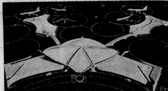
JETPORT-Suggesting flight itself is this model of the new 12-million-dollar Trans-World Airlines passenger terminal to be built at New York International Airport. To be completed in 1960 the thin shell concrete structure will have a main waiting area in the center, with baggage and ticket areas located in the two wings. Glass-ceilinged passageways with moving sidewalks will speed travelers to the boarding areas at upper left and right where 14 jet airliners can be posi-
