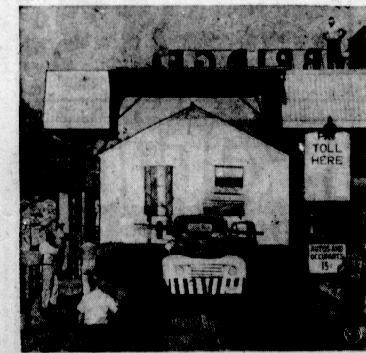
CHEAP AT TWICE THE COST —You can move your home across the Mississippi River for just 60 cents, provided you go by way of the Eads Bridge, and, if it will fit through the toll gate. The Crown Construction Co. of St. Louis found this out when they moved this home to East St. Louis, Ill. Workmen removed part of the eaves of the house and then they were held up by the toll collectors. The collectors checked their books, but couldn't find a specific charge for a house in transit. So they charged them four times the auto cost and sent them on their way.
