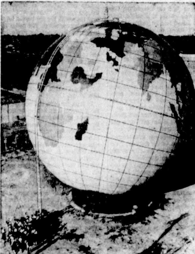
WORLD'S LARGEST WORLD —A "world" full of gas dwarfs spectators at Savannah, Ga., where the globe, said to be the world's largest, does duty as a gas storage tank for Savannah homes. The sphere is made of steel, measures 60 feet across 189 feet around the equator, and stores 600,000 cubic feet of gas for the South Atlantic Gas Co. At lower left a Girl Scout teaches a geography lesson.
