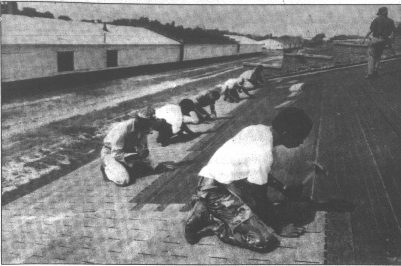
JOB CORPS TRAINEES —At the nation's largest Job Corps center in Morganfield, Ky., Derrset Brown, foreground, of Charleston, S.C. joins other trainees in a roofing class. They
