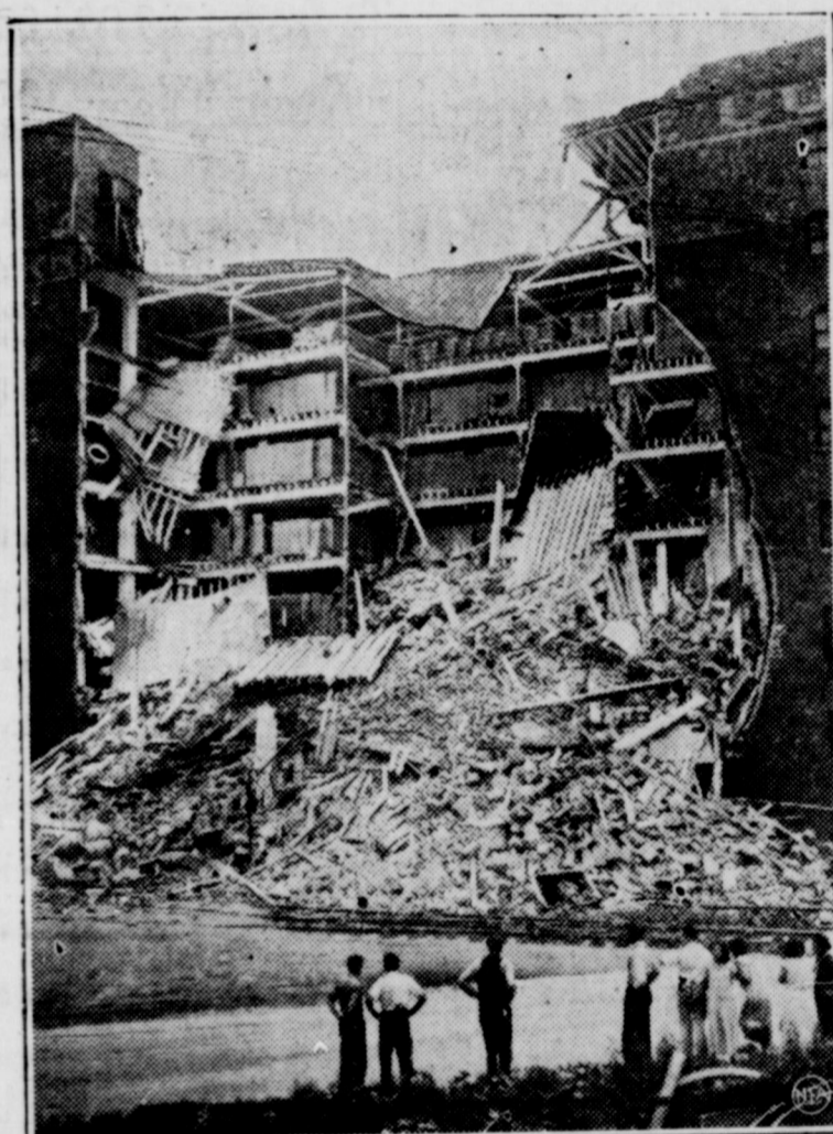
Here is one relief problem that presents a colossal job of "digging out from under," in the collapse of a seven-story Chicago warehouse where the government had stored hundreds of tons of food for the needy. The structure was packed to capacity, as the shelves along the wall still standing show. When one wall crumbled, thousands of barrels and sacks of foodstuff and boxes of canned goods were buried in the walls and vibration of switch engines nearby to have caused the debris. A fire several years ago is believed to have weakened the collapse.
