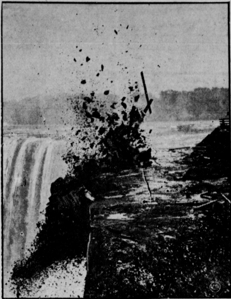
Niagara's roar was momentarily challenged as this man-made blast tore a 5000-ton slice off Table Rock at the Canadian tip of Horseshoe Falls and sent it crashing into the gorge below. Fifty thousand holiday visitors watched spellbound as a second blast reduced the ledge, often called "Honeymoon Point," to half its former size. The dynamiting was undertaken to guard against possible rock slides from a crack extending 200 feet along the table.
