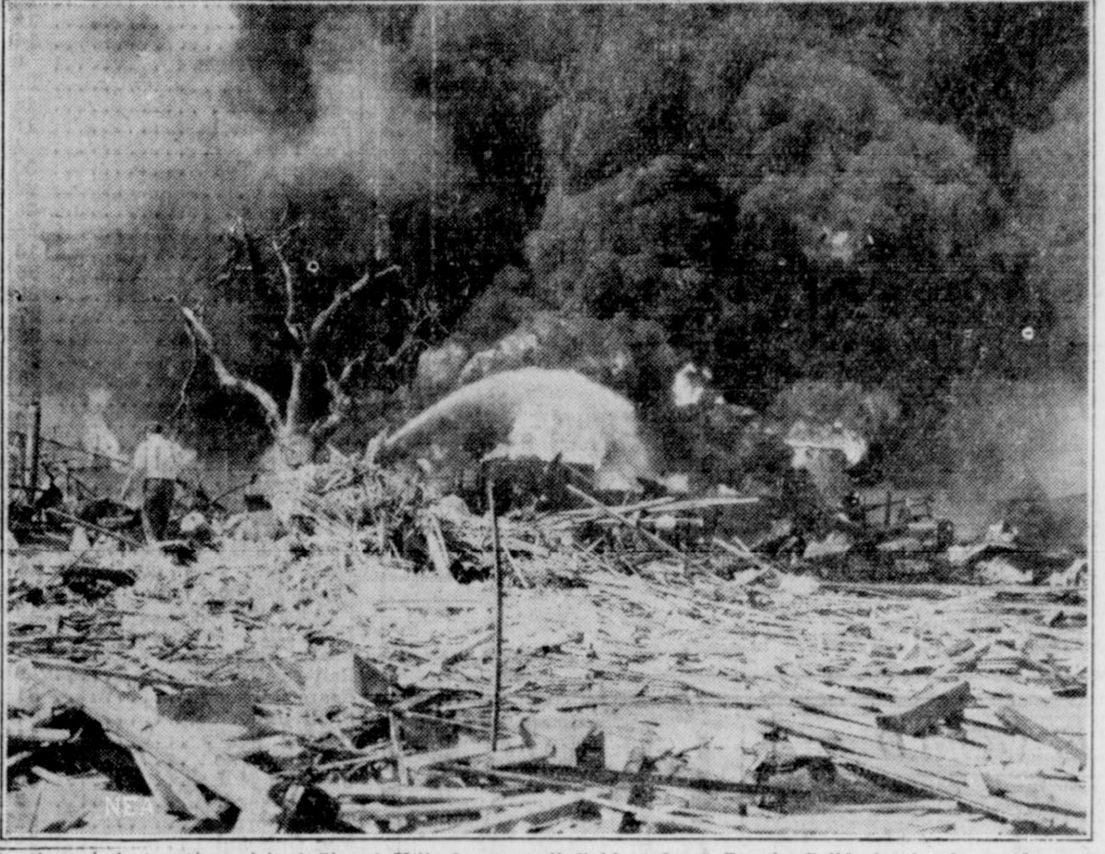
Death and destruction visited Signal Hill, famous oil field at Long Beach, Calif., in the form of an explosion and fire which killed possibly 20 persons and injured many more.
