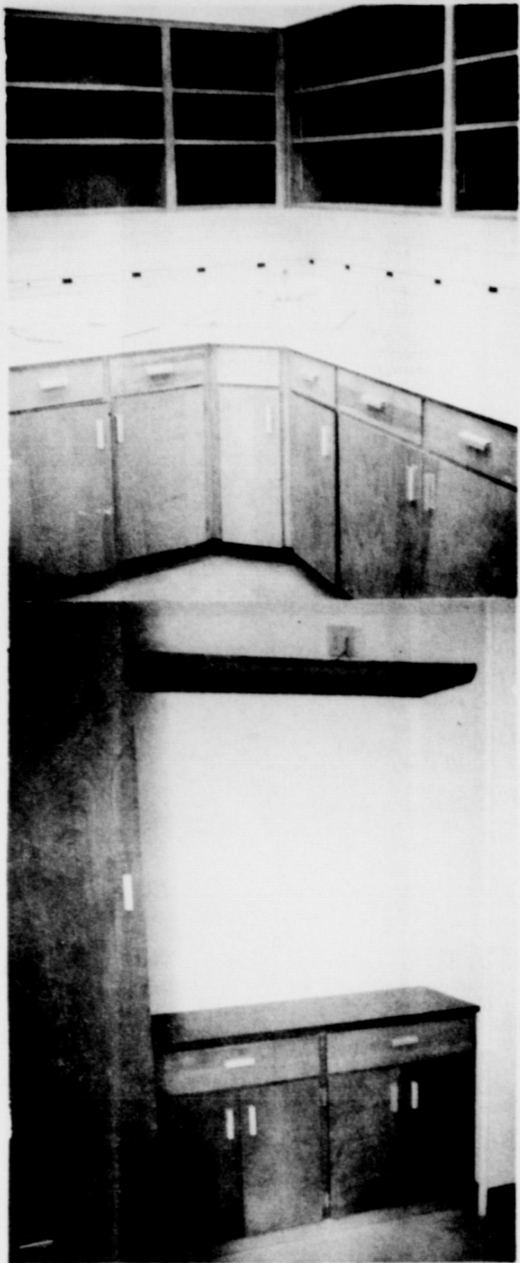
Nearing Completion: Shown here are the built-ins in the sterilizing room and the cabinets in one of the patient rooms. The rooms of the hospital are all painted and the workmen are in the process of laying the floor tile and installing the bathroom fixtures and the kitchen still lacks the cabinets. Some of the sidewalks and concrete work is in the process of being completed.
