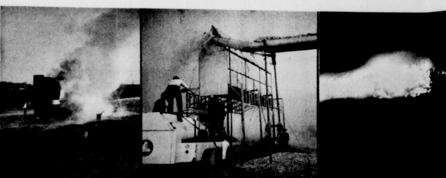
FIVE FIRES: The firemen were put to work extinguishing five fires over a three day period. The first fire was at the Highway barn north of town Monday morning. The Asphalt heater (left) caught fire while it was being prepared for use. Some water in the pipes was pulled into the tank and caused an explosion which spilled asphalt over the tank. The heater was a total loss with an estimated value of $4900. The fire truck was called to the T & M Gin (middle) Tuesday afternoon and again Wednesday morning. No damage was done at the gin and the burr pile was on fire in both cases. A 4:45 a.m. alarm sent the fire truck to Allison to fight a burr pile fire (right). The fire was first started by a spark from a tractor at 1:00 a.m.; this fire was extinguished to erupt at 3:00 a.m. The gin crew extinguished the 3 a.m. fire and looked out to find the entire burr pile on fire with the wind out of the north; at this time the Wheeler fire department was called. A grass fire burned 1 1/2 acres before it was doused by the department eight miles west of Wheeler on Chuck Hogan's pasture.
