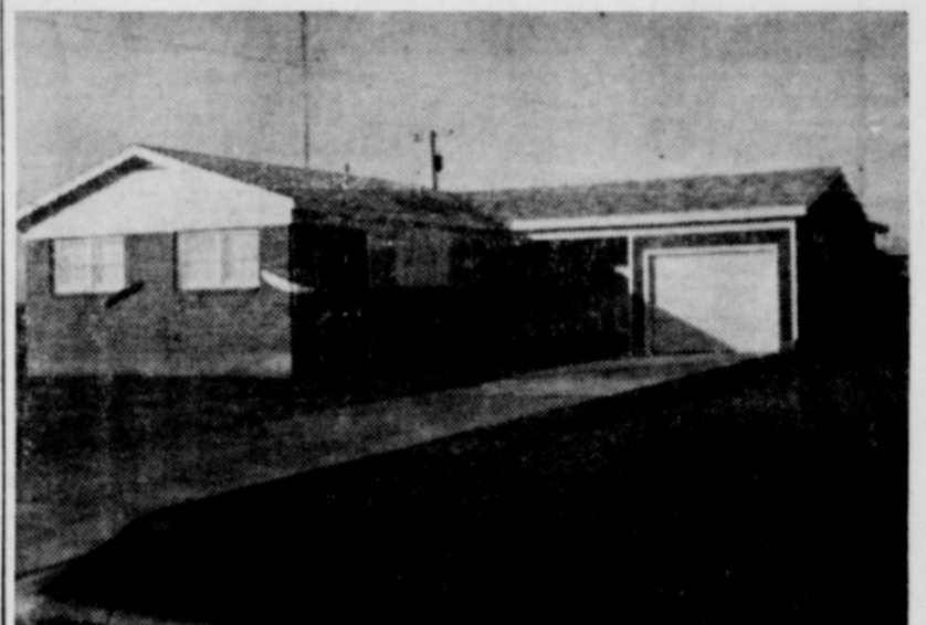
ANOTHER NEW ONE: This is the new home of Mr. and Mrs. Louis Boynton located on the south end of Main Street. The Wheeler Lumber was the supplier and Eli Sabbe, the builder. The Boyntons will move into the new home sometime this week.
