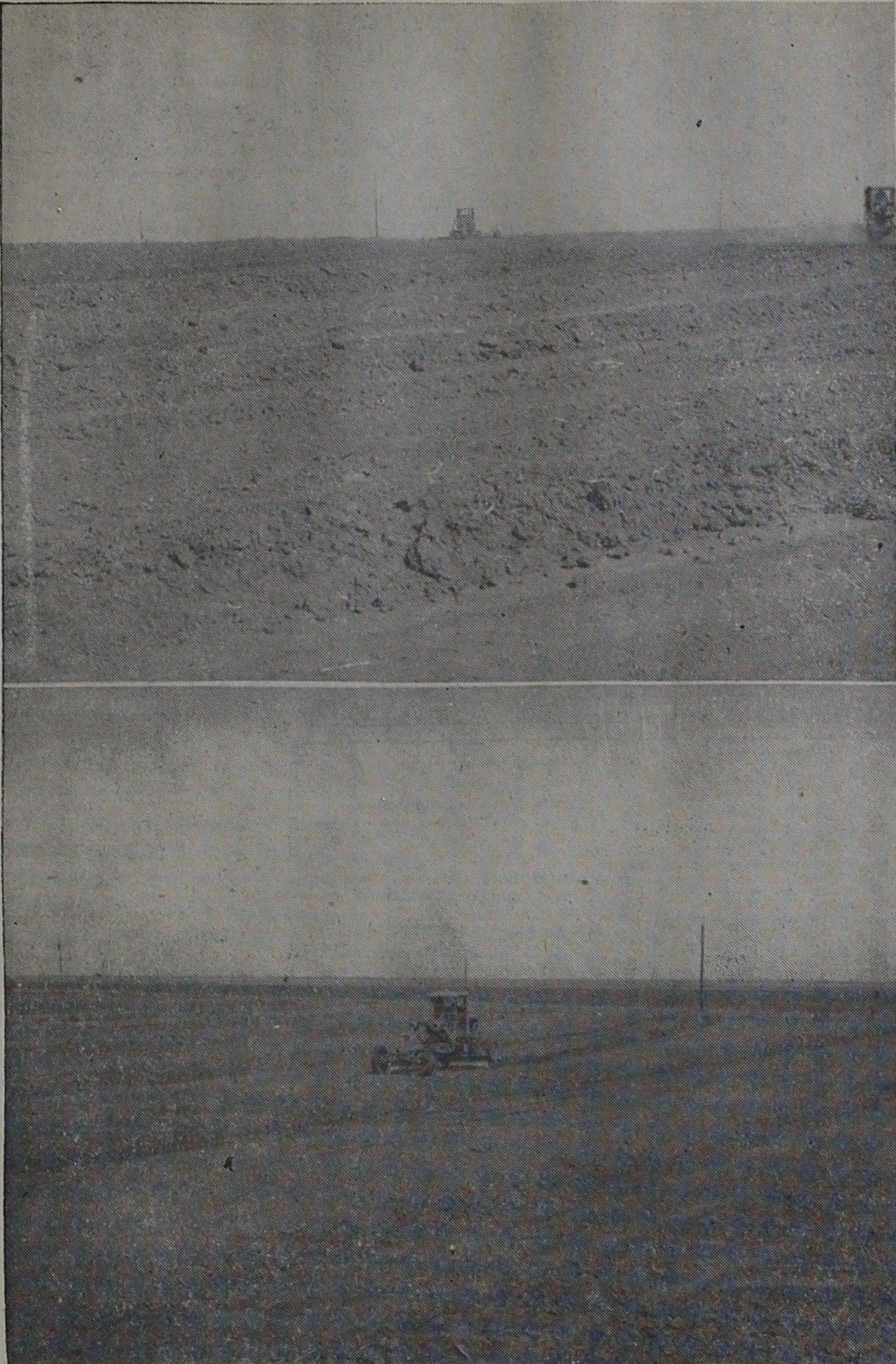
BENCH LEVELLING —These photos were made by SCS technicians while bench levelling work was going on south of Black on the Nelson Coon farm. The top picture: Two motor graders were at work building borders which are parallel and follow the contour of the field. Lower photo: Another view of the field, as a grader levels pan between borders, pulling surplus soil down slope of field. Upper right photo: An uphill view of the waterway which will be grassed to prevent erosion from run-off water.
