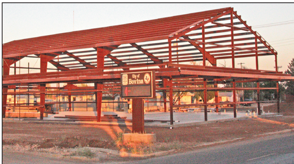
Construction continues on the Bovina Community Center.
