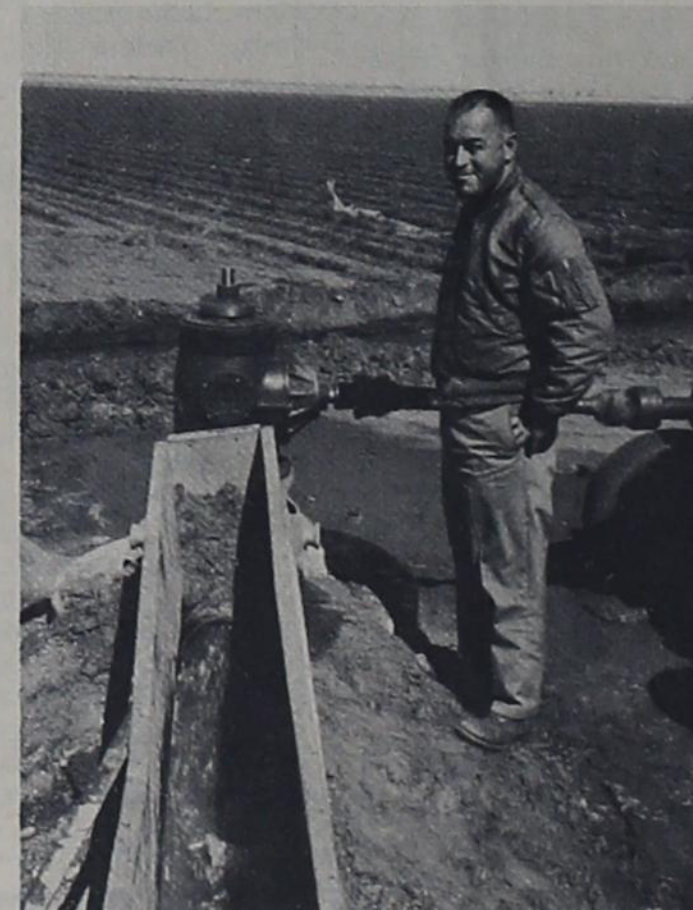
Mark Liethen has a smile of satisfaction for his new 8-inch well, drilled to 405 feet on the Bert Williams farm, located southwest of Texico. The pump was set at 300 feet for a sprinkler system. This is the eighth well drilled in the past four years for Williams by Watts Machine & Pump Company, Inc.
