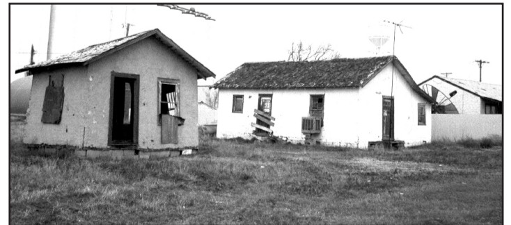
Structures in the 500 block of Avenue A. Houses will be used for fire department practice.
