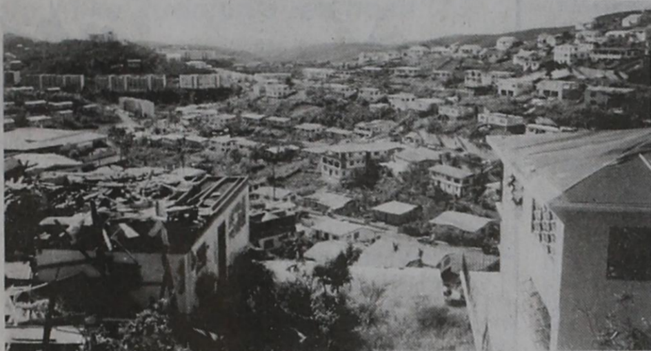
This is just one residential area that we saw that was starting to rebuild after the hurricane. Tarps cover most of the roofs, or what use to be roofs on most of the houses. The family home in the foreground, left, lost everything in the hurricane, while the home to the right only lost their roof.
