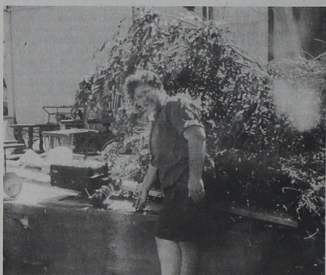
Alta Jesko shows the bolts that held her back porch to its foundation before last week's storm moved the porch to her front yard.
