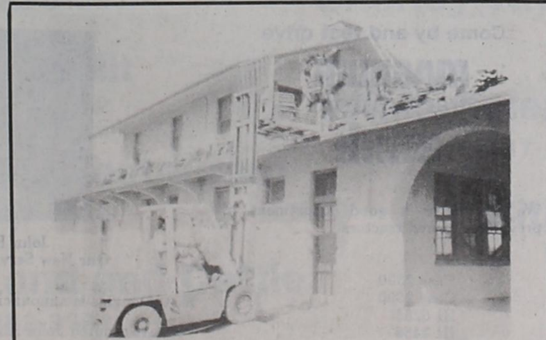
Demolition of the old Santa Fe station in Texico begins.
