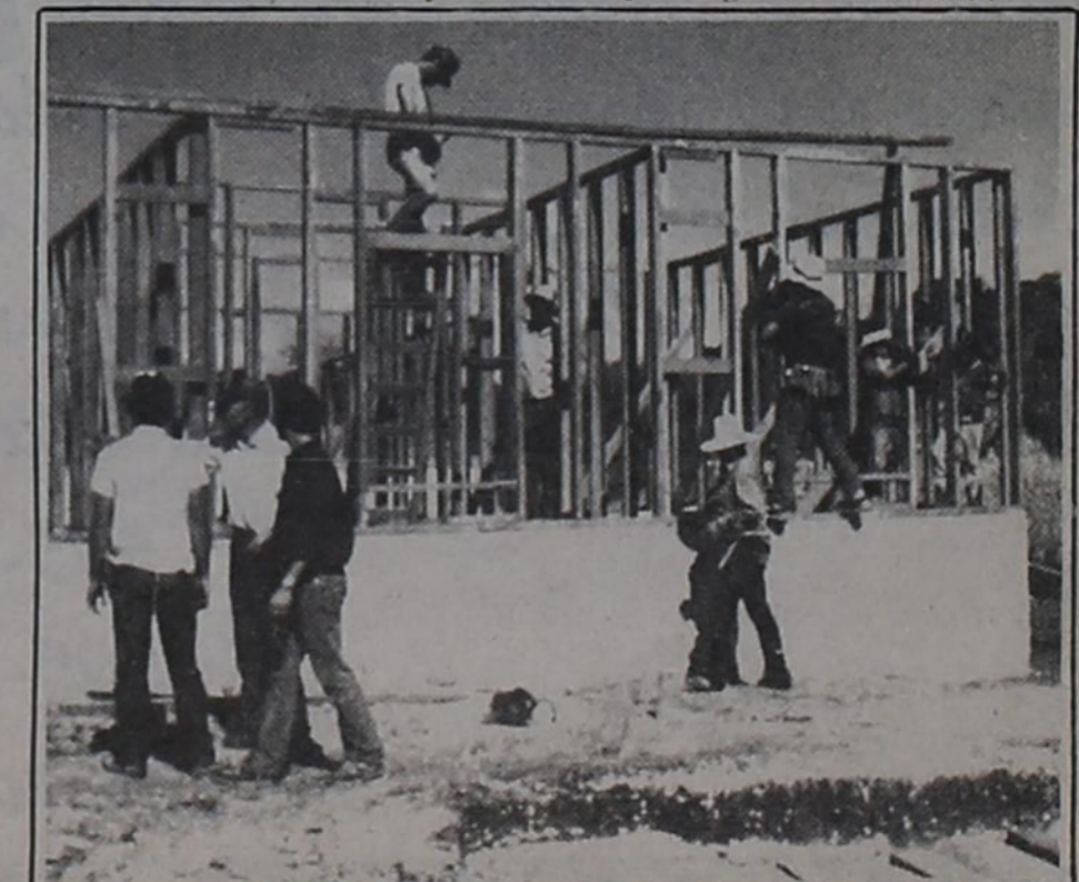
Workers erect the new cafeteria.
