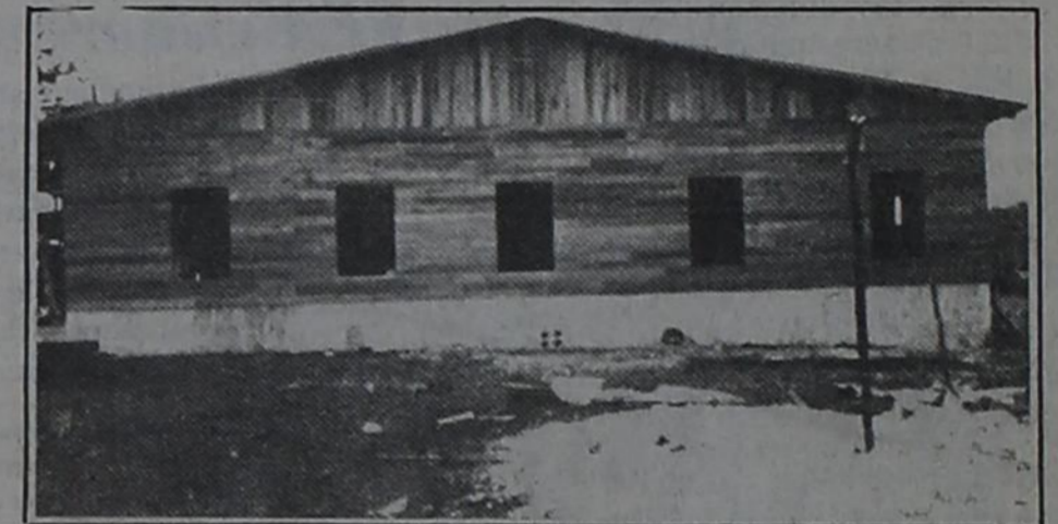
The new cafeteria.
