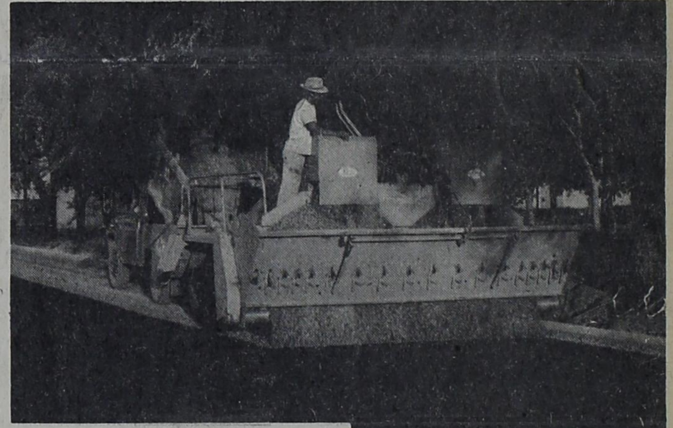
Workmen put finishing touches on one of new paved streets
