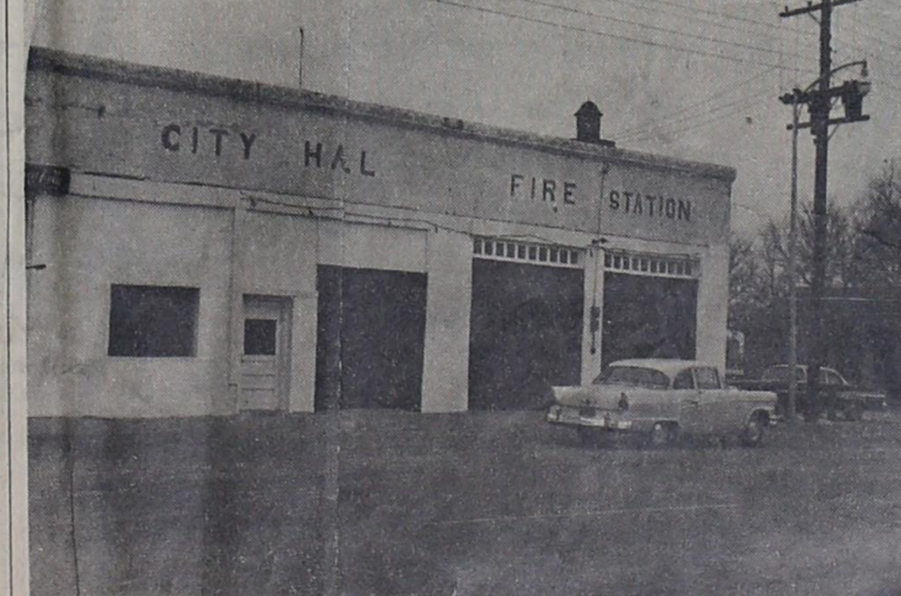
A NEW LOOK--Texico town hall has recently been remodeled. Included in the improvements were new paint inside and out, modernizing of the main office, addition of a garage for a new truck which the fire department scheduled to get, and more storage space.
